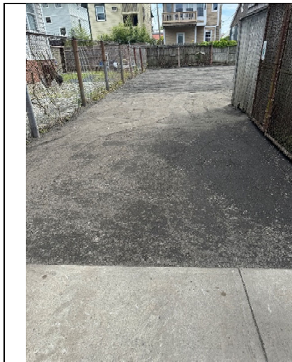
Typical view of finished cap.
