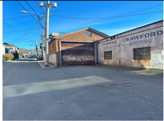
View of temporary cap area.
