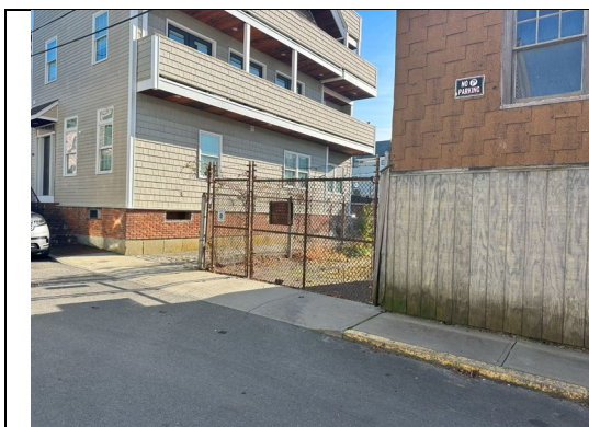
View of locked gate.
