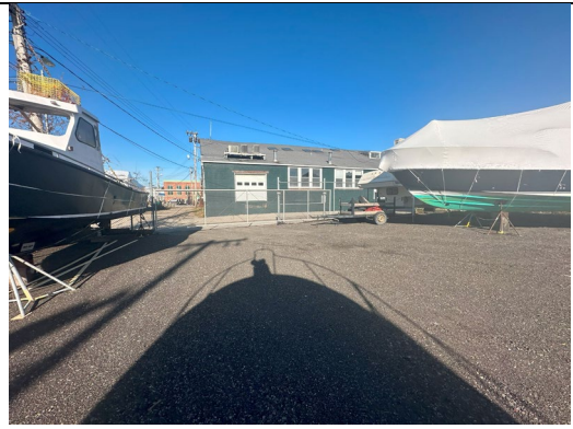
View of temporary cap area.
