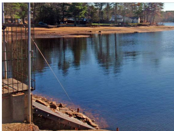
Outlet structure at Keech Pond (Glocester, left) lowers the lake water level exposing docks (right).
